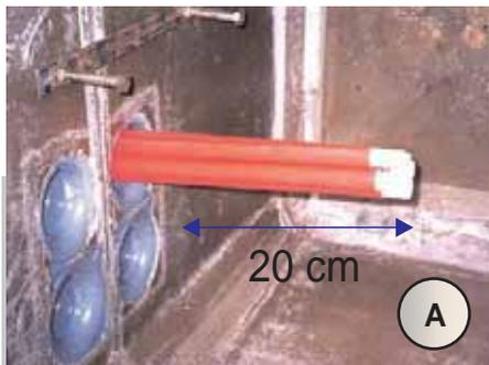
Insert the COD into the MH or HH entry hole. The sub-ducts shall protrude outside the hole by approx. 20 cm.
