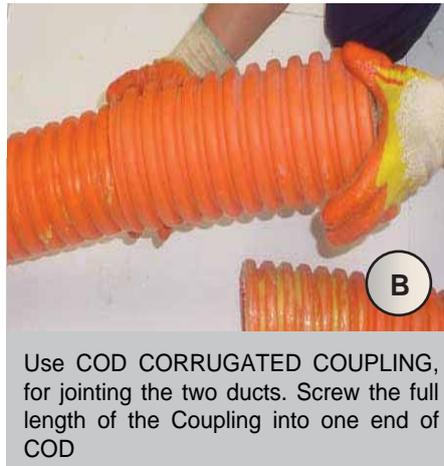
Use COD CORRUGATED COUPLING, for jointing the two ducts. Screw the full length of the Coupling into one end of COD
