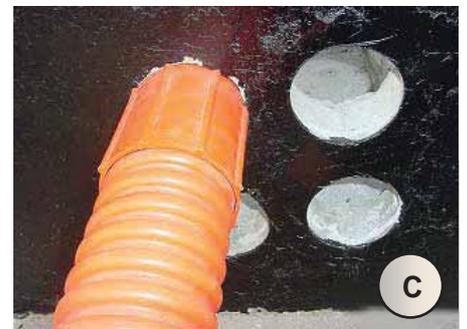
Insert the COD duct into the MH or HH
