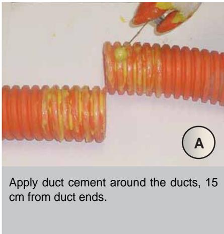
Apply duct cement around the ducts, 15 cm from duct ends.
