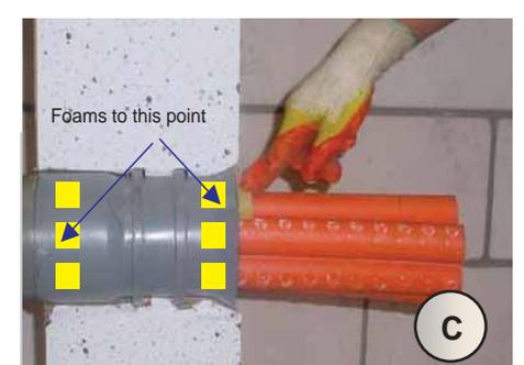
Insert foams near the hole's opening.
