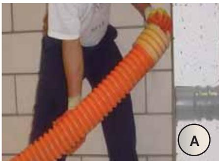
Pull the COD duct up to the manhole or
