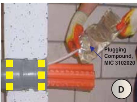
Prepare the Plugging Compound and inject between the foam barriers.
