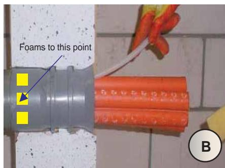
First, insert foams around the spaces at one end of the duct terminator.
